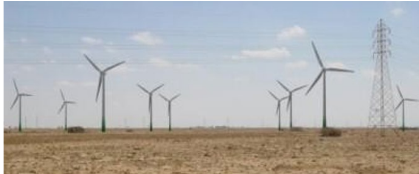
Figure (3) Wind farm in Darnah
