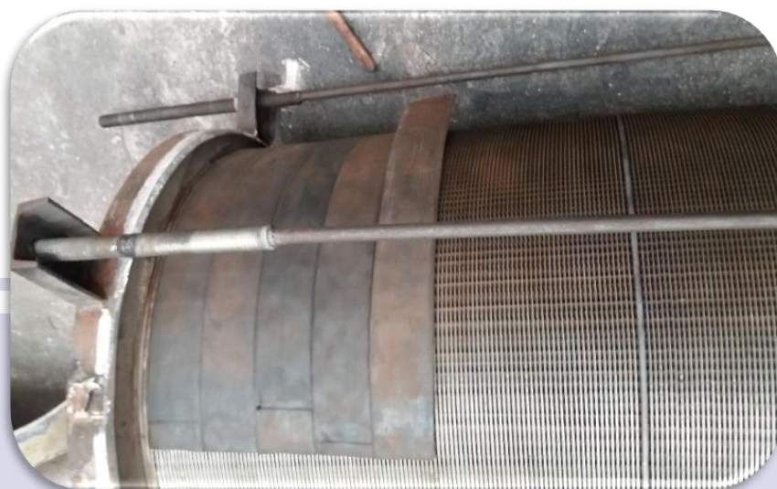
FIGURE No (8)- Recovering exchanger with its jacke
