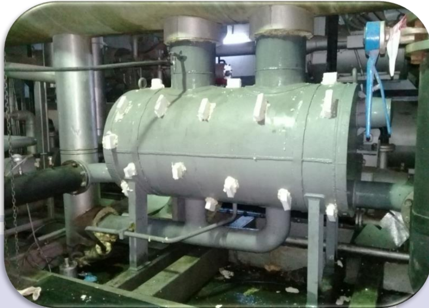
FIGURE No (14) - Re-isolate the evaporator body (cover supporting)
