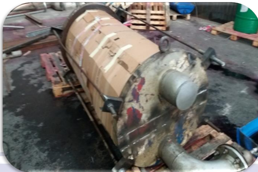
FIGURE No (4) - Isolate the evaporator area against the cutting
