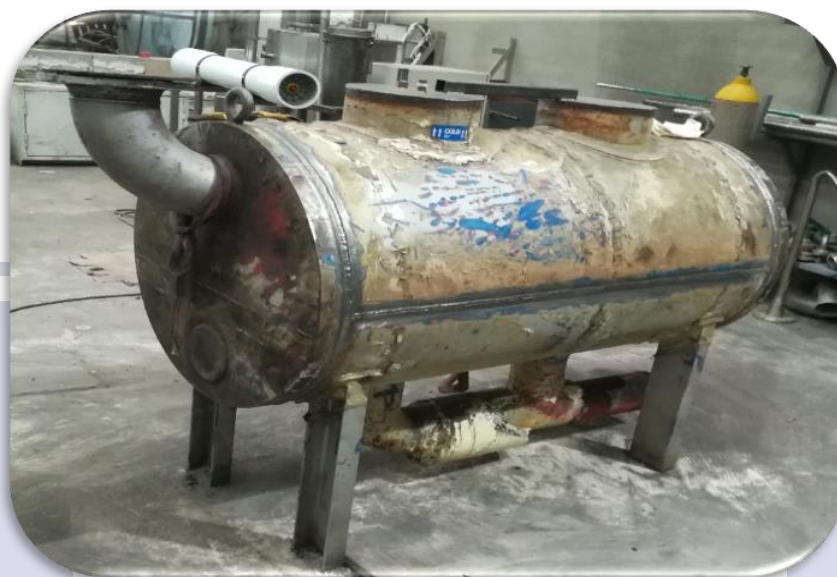
FIGURE No (10) - Assembly the evaporator inside its case
