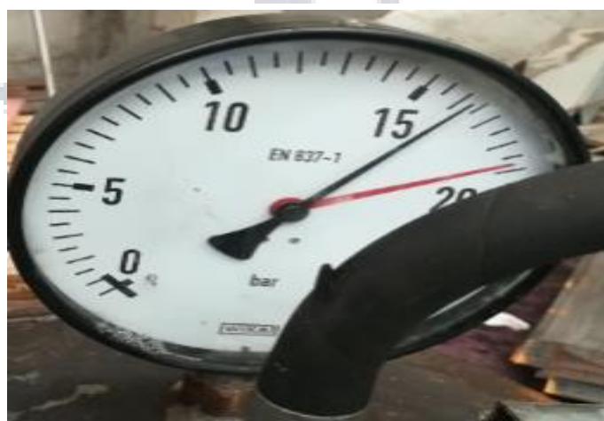
FIGURE No (9) - Pressure test 16 bar
