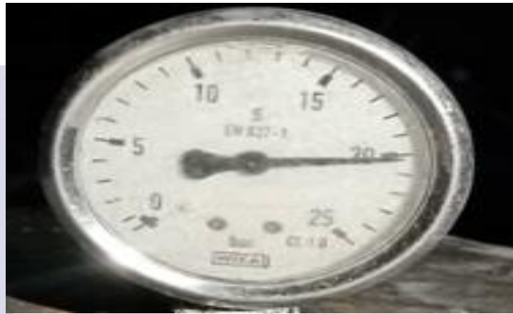
FIGURE No (6) - Pressure test 20 bar
